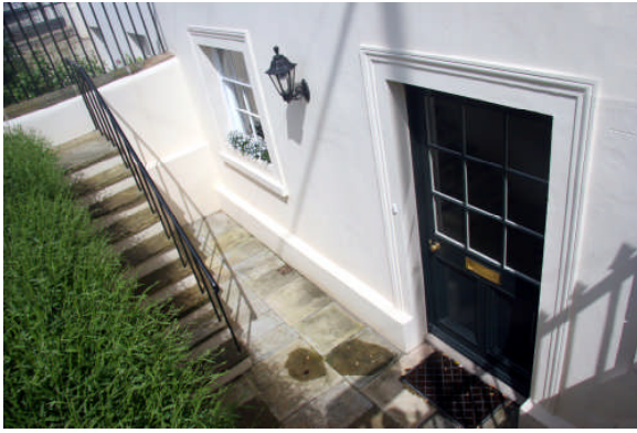
Fine restoration of façade and basement, Dale Street
