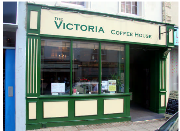
New shop front, Warwick Street
