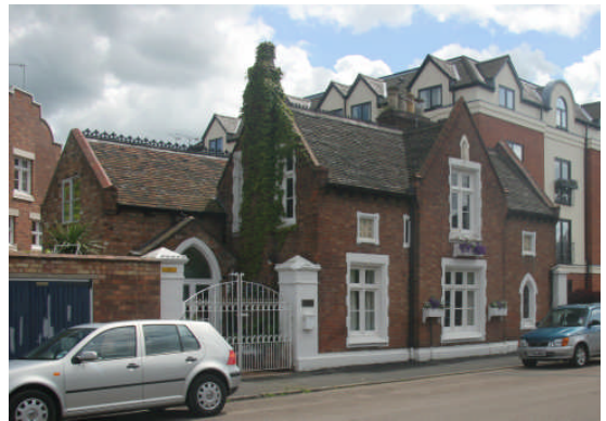
Careful restoration and matching new wing, Farley Street
